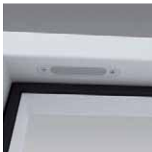
Detail 4 Monitoring contact
