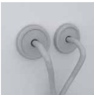
Detail 3 Cable feed-through
